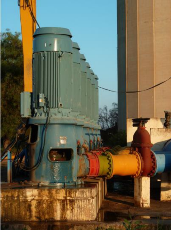
Situation before replacement
